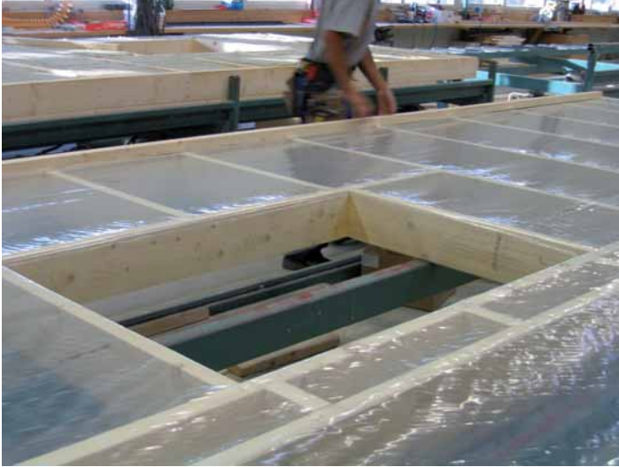
Figure 5.8 Prefabrication of outer walls.
