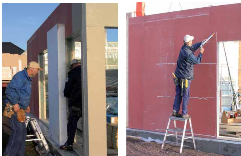
Figure 5.14 Polystyrene glued on the gypsum board.
