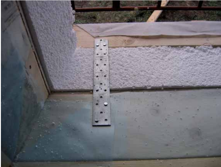
Figure 5.19 Nailing plates in window openings.
