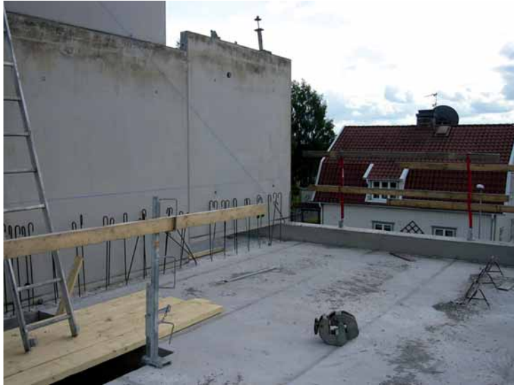
Figure 2.3 Concrete inner walls cast on site.
