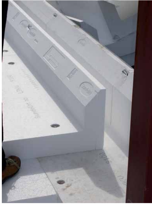
Figure 3.7 Foundation construction insulation.
