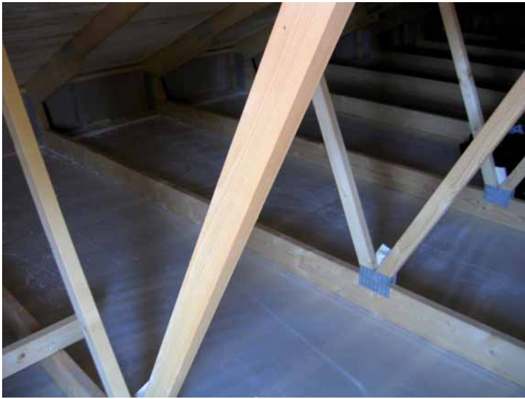
Figure 4.12 The attic, before the insulation was put in place.
