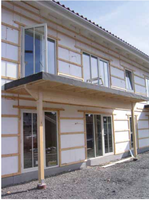
Figure 4.10 Walls covered by polystyrene.
