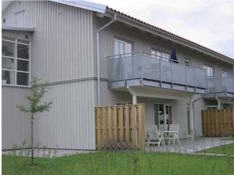
Figure 2.5 The apartment buildings in Frillesås.
