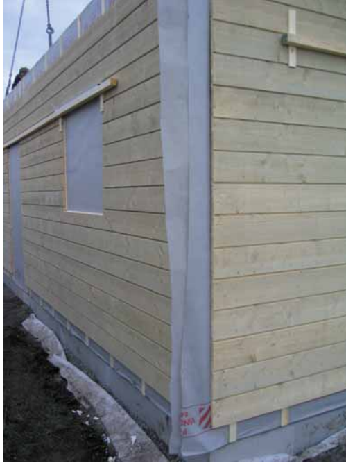
Figure 5.18 Lowest wooden panel detached to facilitate the mounting process.
