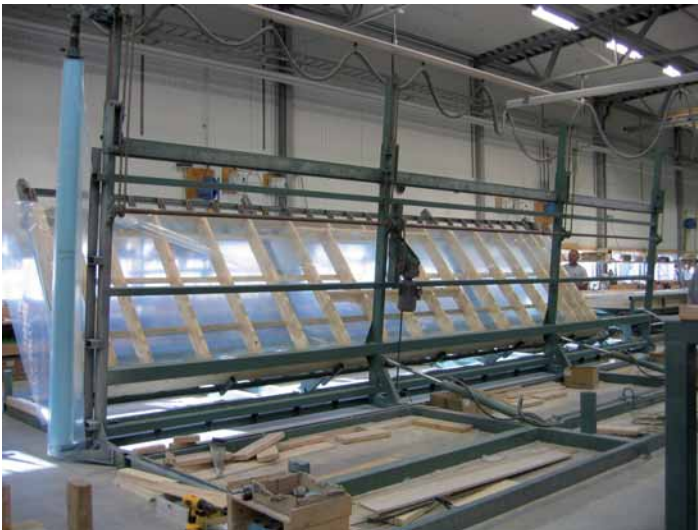
Figure 5.9 Other side of outer wall.
