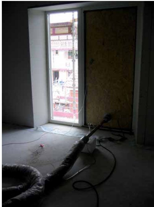
Figure 4.16 Wooden board mounted for airtightness measurement.
