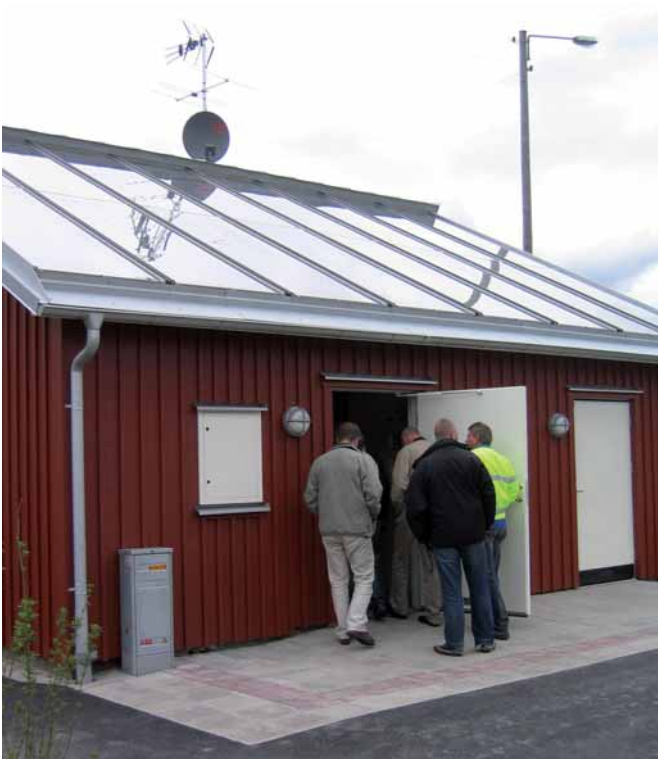
Figure 2.10 Solar collectors on the roof of the apparatus building
