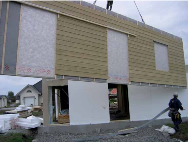
Figure 5.17 Outer wall slab is mounted.
