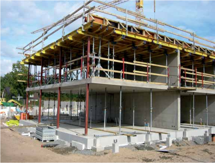
Figure 3.8 Concrete construction cast on site.
