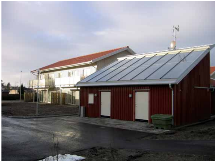
Fig 4.6 Solar collectors on the roof of the apparatus building.
