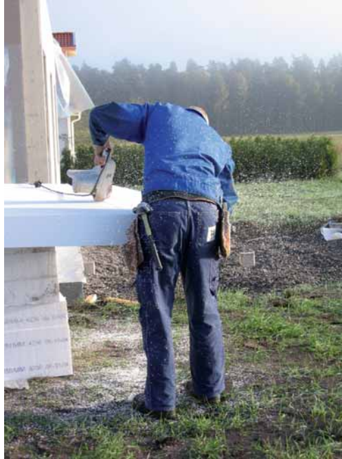
Figure 5.15 Polystyrene sawn up on site.
