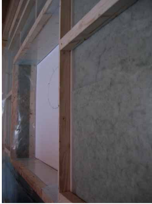
Figure 5.12 Wooden frame construction for installations.
