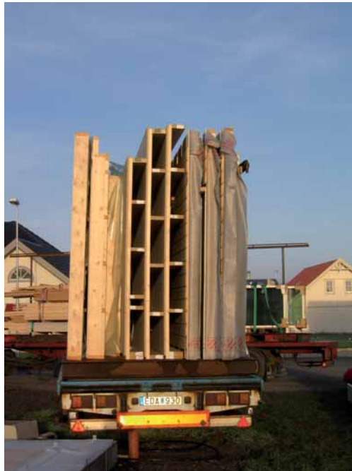
Figure 5.7 Wall panels transported to the site.
