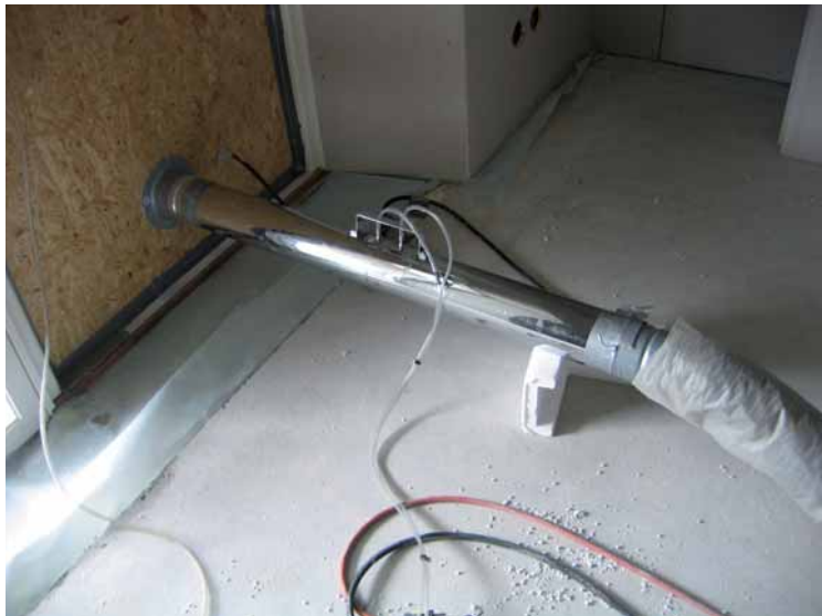
Figure 2.9 Measurement of air leakage.
