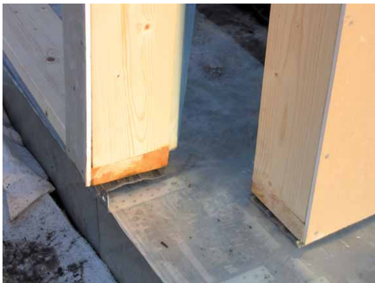
Figure 5.13 Moisture protection of wooden beam construction.
