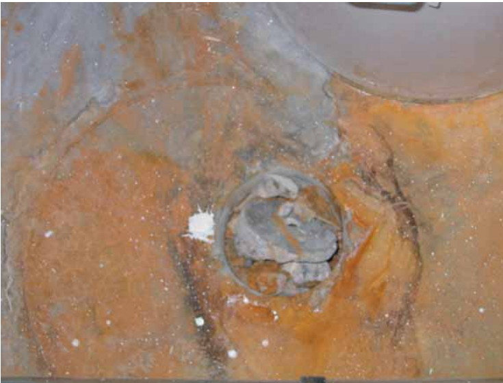
Figure 5.23 Measurement of moisture content in concrete slab.
