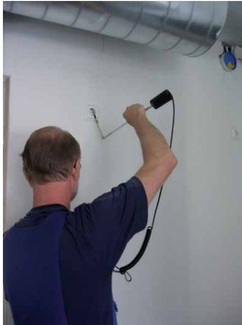
Figure 4.20 Measurement of air leakage through electrical sockets.
