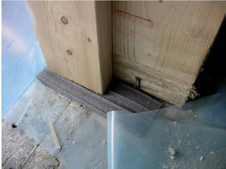
Figure 4.11 Moisture protection in the wooden sill construction.
