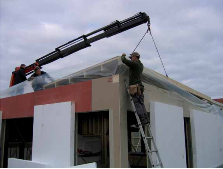
Figure 5.16 System of beams mounted on top of the walls.
