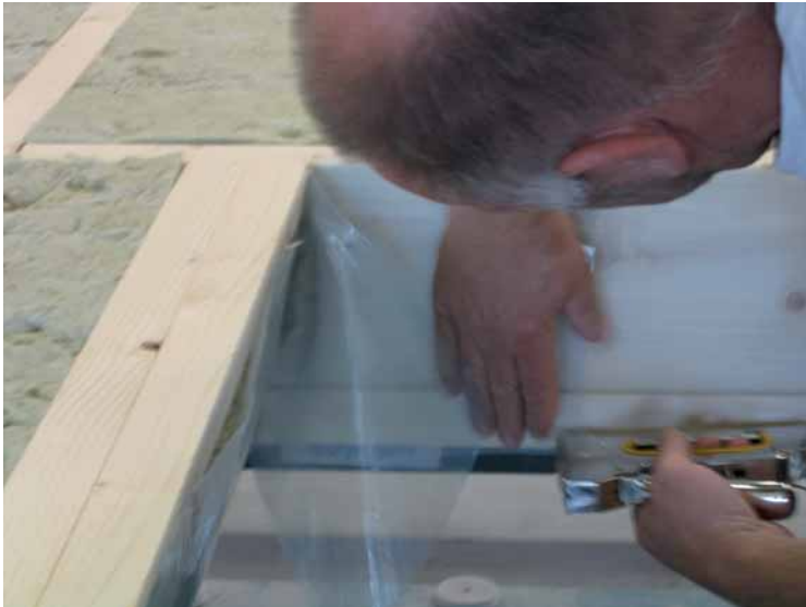
Figure 5.10 Mounting of plastic foil.
