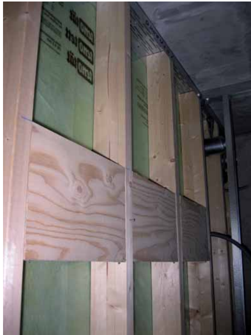
Figure 3.10 Space for installation.
