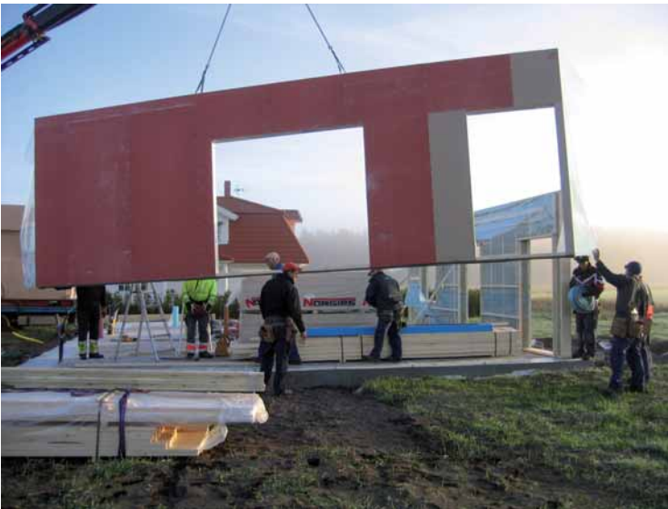
Figure 5.11 Mounting of inner slab.
