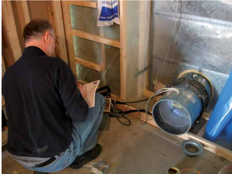
Figure 5.22 Measurement of airtightness.
